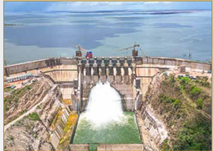
Julius Nyerere Hydropower Plant
