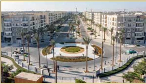
Mivida Project - Mixed Use Boulevard & Site Works, Cairo, Egypt
